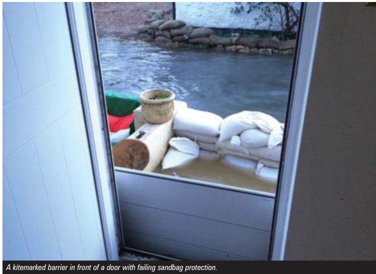
A kitemarked barrier in front of a door with failing sandbag protection.
